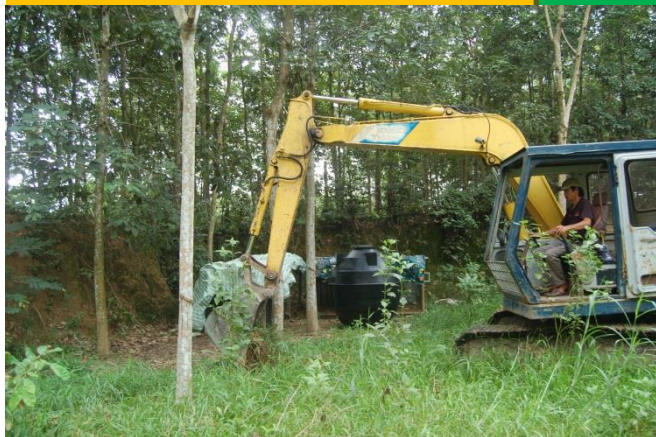
Photo 3: An excavator is digging a hole to bury the septic tanks
