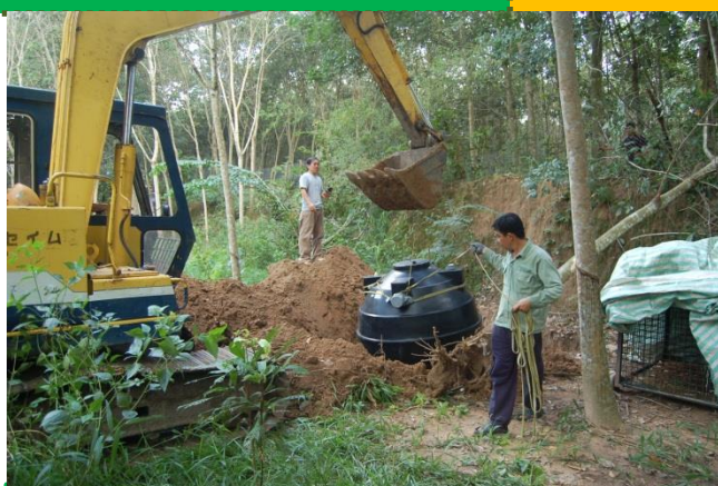
Photo 4: The excavator is lowering the tank into the hole.
